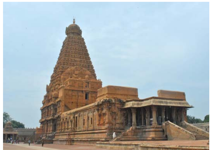
View from south east side
